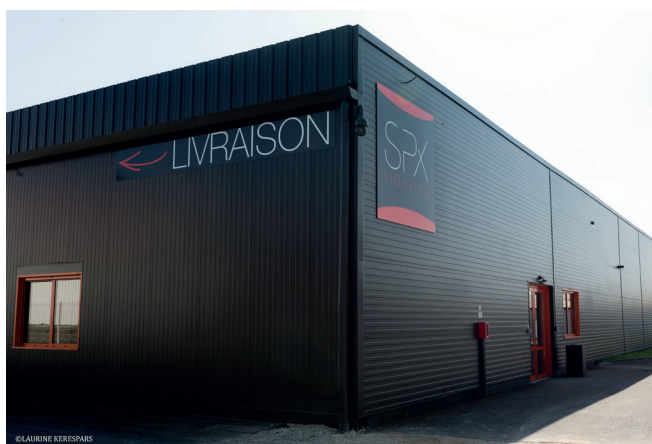
Site de Production SPX Lighting - Issoudun - France
