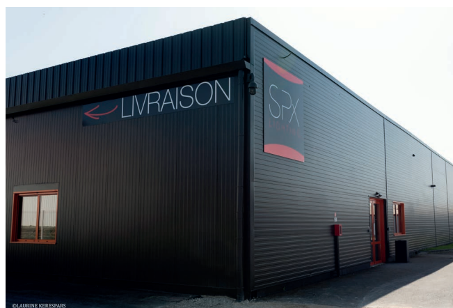
SPX Lighting - Issoudun - France
