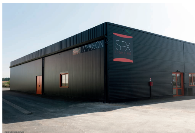
Factory SPX Lighting - Issoudun - France
